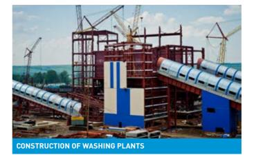
Another important development in 2011 was the start of construction on a second washing plant (Kaskad-2), which the Company plans to complete in the fourth quarter of 2012. The plant will have capacity of 4 million tonnes, two times more than the plans presented to participants in KTK's IPO in 2010. The plant will simultaneously use steeply inclined separation and dense medium gravity separation, which is an innovative technology in both Russian and globally.
